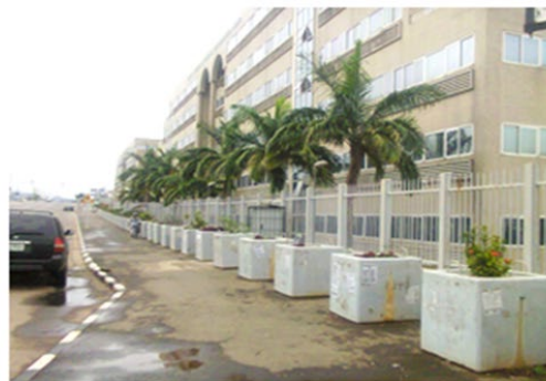
Plate VII: Metal fence with visual continuity aids surveillance. Engineered planters are used as vehicle barrier to deter use of bomb-laden vehicles to target the building (Ministry of Finance, Abuja). Photo credit: Samuel Ebong
