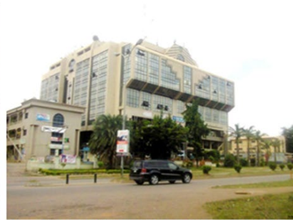
Plate II: A building design with windows that allow natural observation of areas outside the building thereby increasing deterrence (AP Plaza, Wuse II, Abuja). Photo credit: Samuel Ebong
