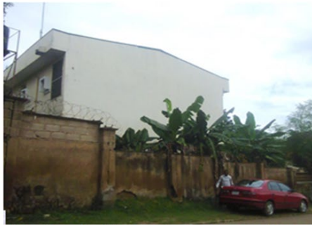
Plate I: A blank wall creates surveillance shadow that could reduce deterrence and compromise security (Residential Building, Wuse II, Abuja). Photo credit: Samuel Ebong
