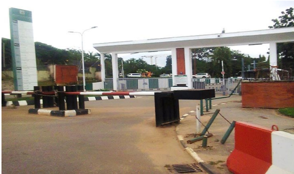
Plate III: Drop arm security barricade for access control is positioned in front of the gate as a vehicle arrest system (Federal Capital Development Authority Complex, Abuja). Photo credit: Samuel Ebong
